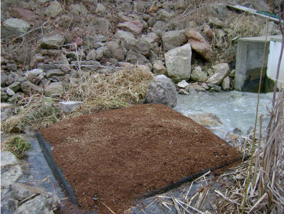
A Newly Installed BioSwale
